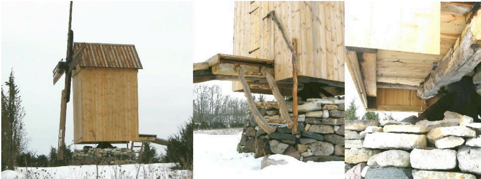
The restored postmill in Viltina is built around 1780. Since its establishment, it has changed its location 3 times. The Viltina Villem's postmill has been in its position now over 130 years and still belongs to the same owners family. Its construction and exterior has been restored, mechanisms are conserved at the moment.
